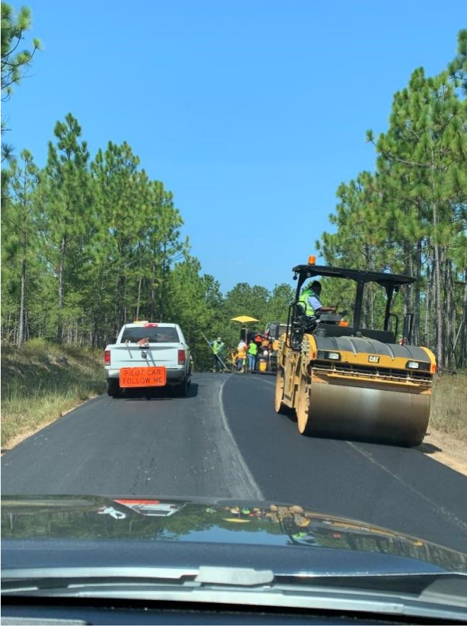
Paving in Progress --
