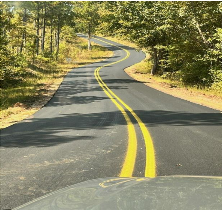
Paving complete – including yellow stripes !!
